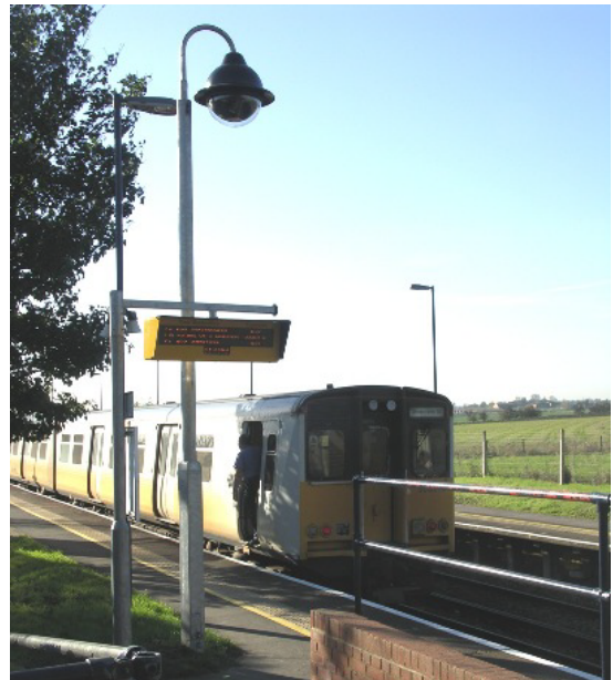
The new CCTV installation at Kemsley Station can monitor both platforms
